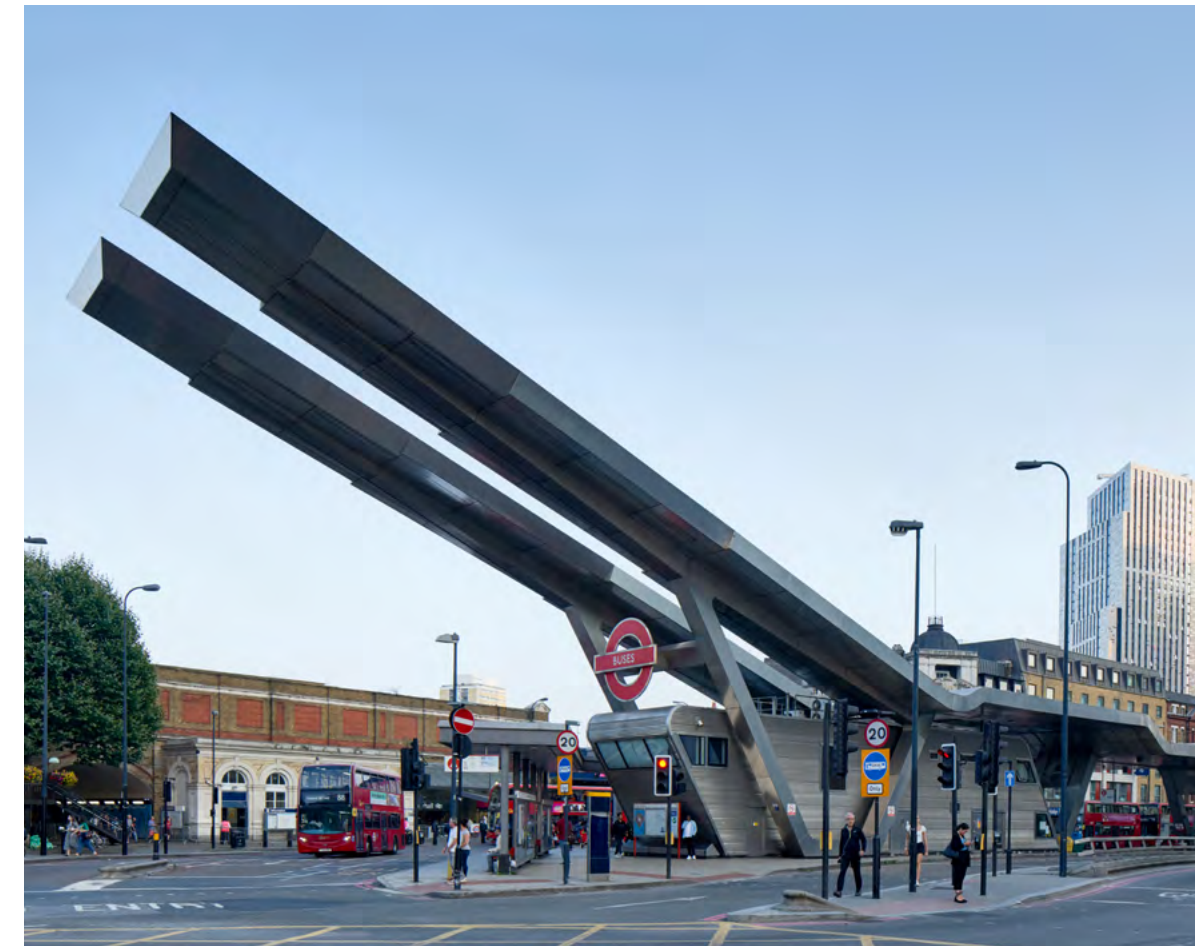
THE BUS STATION WAS DESIGNED BY ARUP ASSOCIATES. IT INCORPORATES TWO CANTILEVERED ARMS THAT CONTAIN 167 SOLAR PANELS.
