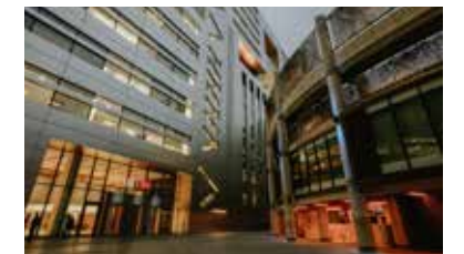
UBS Main Office
